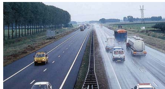
Figure 1: Drainage with an open graded asphalt wearing surface versus a densely graded asphalt surface [Jong 1999]
