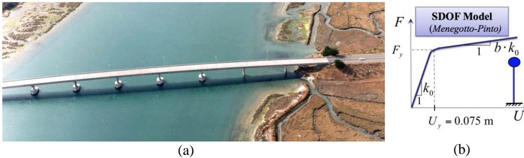
Figure 4: Humboldt bay middle channel (HBMC) bridge (courtesy of Caltrans): (a) isometric view, and (b) simplified nonlinear SDOF model to represent the longitudinal nonlinear response behavior of the bridge
