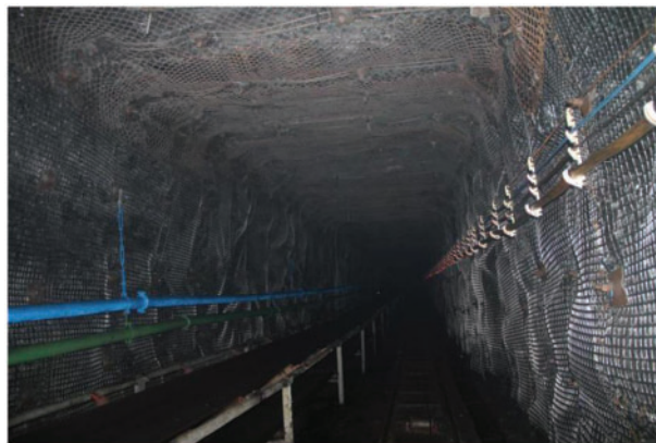
Figure 16: Actual effect of roadway support
