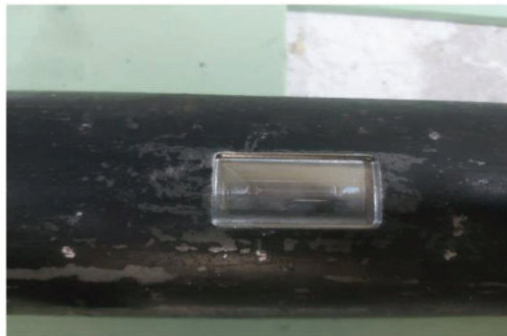
Figure 5: Defect created on the tank
