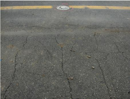
Figure 5: Rutting and alligator cracks near the centerline
