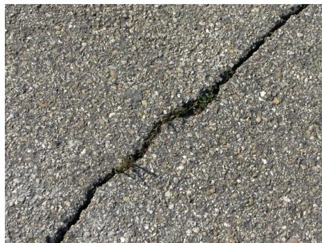
Figure 8: Detail of Fig. 7 and polished worn aggregates on the taxiway surface
