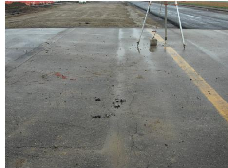
Figure 6: Behavior of the taxiway after a rain: the undrained water staying inside the wheelpaths channels created by rutting, possible cause of hydroplaning, is well evident; wheelpath cracking caused by traffic loads is also evident in the upper left corner
