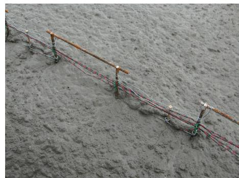
Figure 19: Concrete flowing through the strain-gauges during concreting
