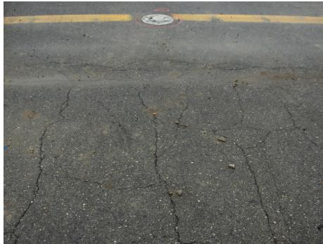
Figure 5: Rutting and alligator cracks near the centerline
