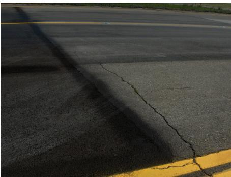
Figure 7: Open cracks with some grass growing inside
