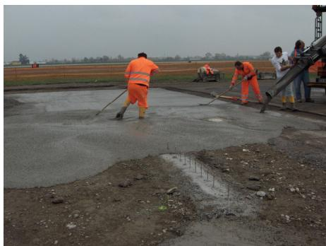
Figure 18: Concreting of Section 2 semi-rigid pavement
