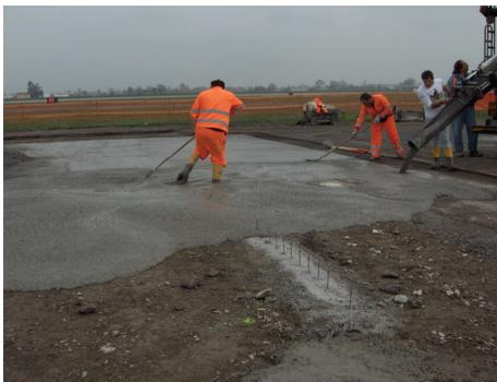
Figure 18: Concreting of Section 2 semi-rigid pavement
