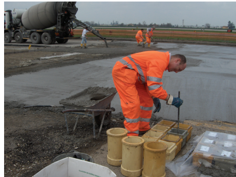
Figure 17: Preparation of cubic and cylindrical specimens while concreting Section 1 semi-rigid pavement
