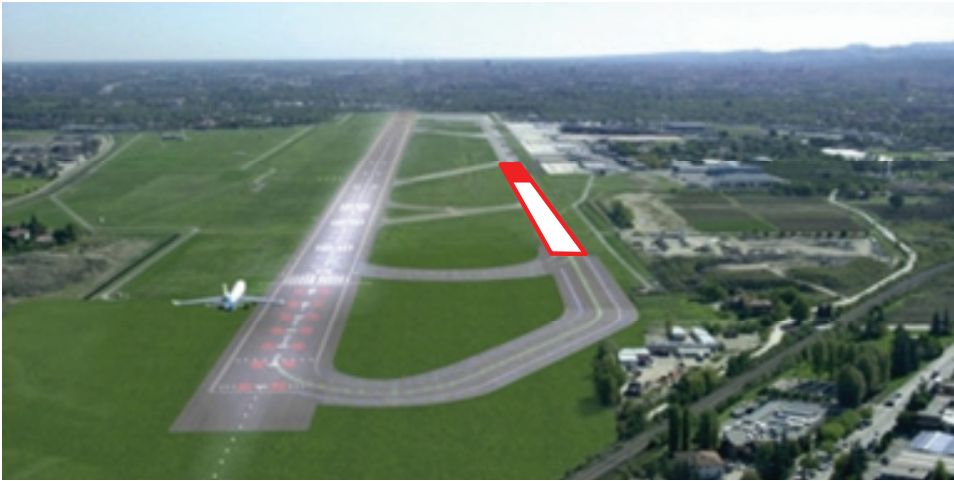
Figure 2: Rehabilitation interview of the taxiway at the Guglielmo Marconi airport of Bologna (Italy): area of the rehabilitation interview boxed in red and experimental segment filled in red
