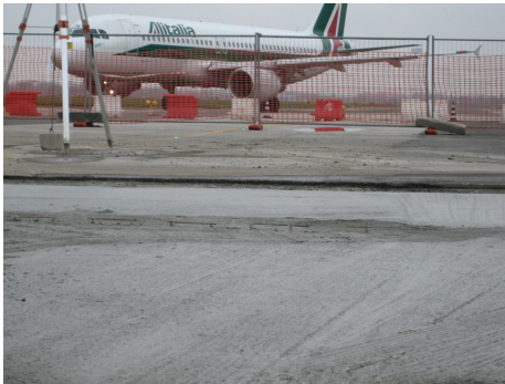
Figure 16: Metallic support after concreting
