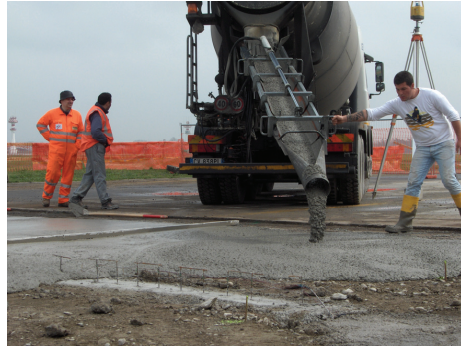
Figure 13: Concreting of Section 2 semi-rigid pavement
