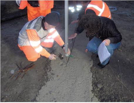
Figure 12: Base of the mobile unit for GPS topographic surveying rested over the metallic support during installation of the metallic support itself
