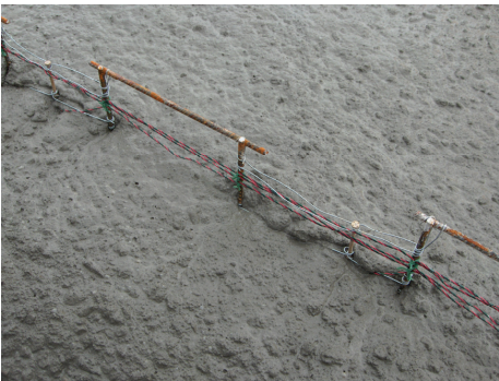
Figure 14: Concrete flowing during concreting
