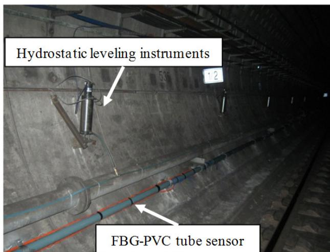
Figure 4: Typical Hydrostatic Level and FBG-PVC tube sensor installed in the tunnel
