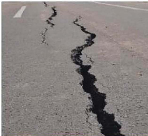
Figure 2: Subgrade cracks
