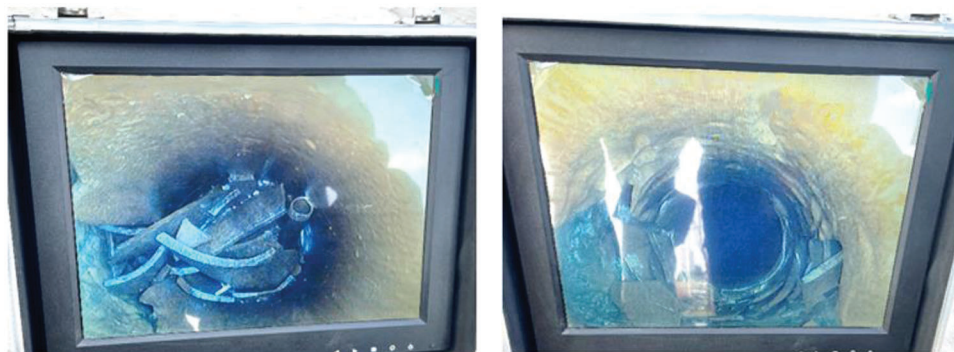
Figure 3: Scanned image of the inner wall of the borehole
