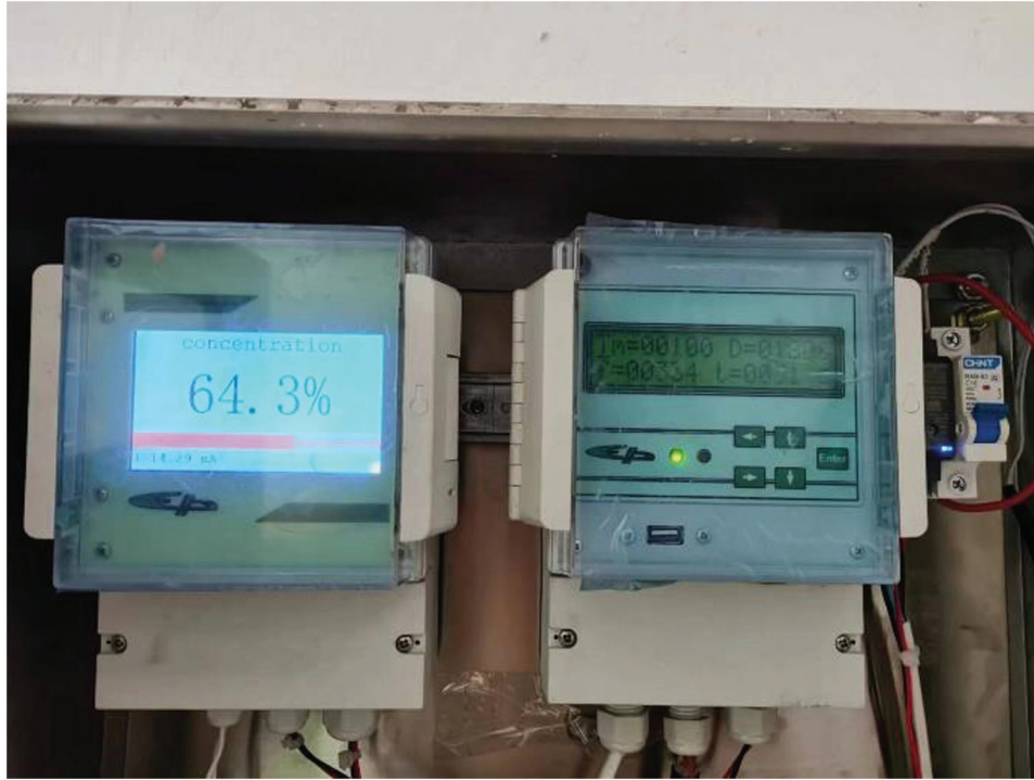
Figure 5: Radioactive density gauge
