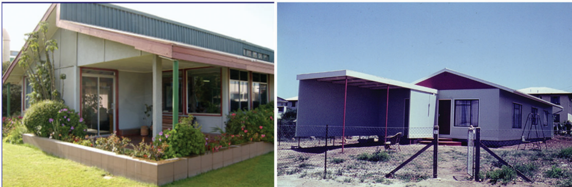
Figure 7: Buildings exclusively built with double walls of tannin-based particleboard. Office building with walls of pine tannin adhesive bonded particleboard 20 years after its construction in Chile (left). Low cost house with walls of mimosa tannin adhesive bonded particleboard immediately after its construction and still standing today in coastal area in South Africa (right)
