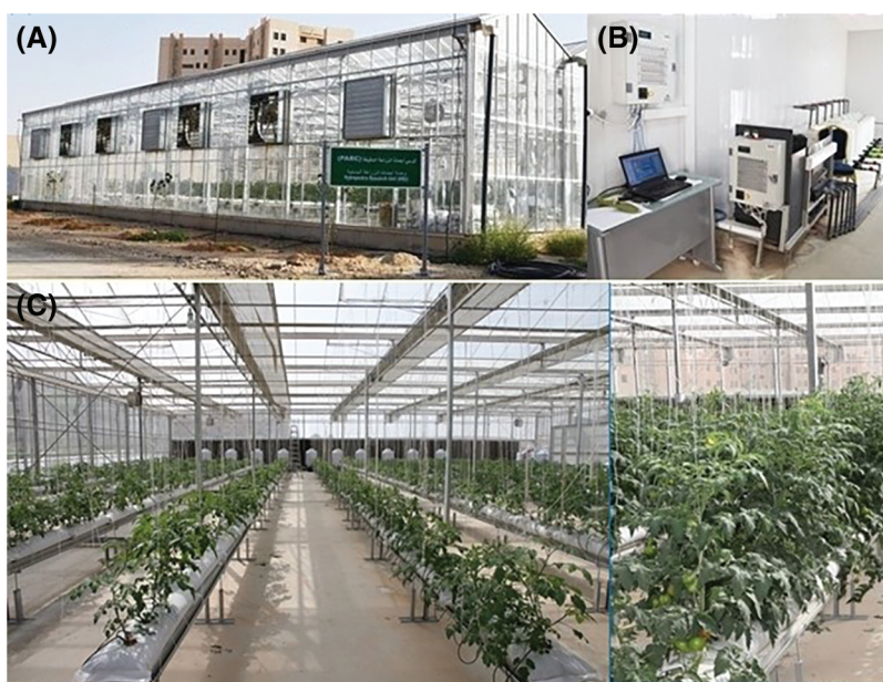
Figure 1: (A) The hydroponic greenhouse, (B) control unit, (C) steel troughs (plant lines) including perlite bags and plants as well as the irrigation system
