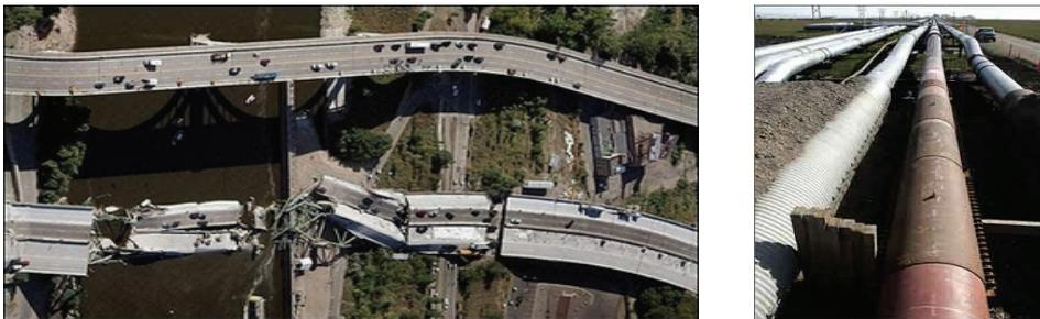
Figure 1: Recent failures resulting from corrosion damage in bridges and pipelines (from USA Today)
