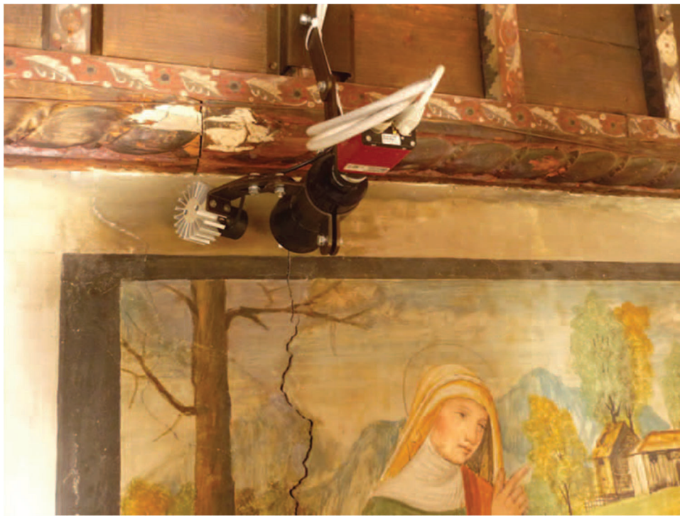
Figure 6: High-definition Optical video camera for nondestructive static monitoring [29]
