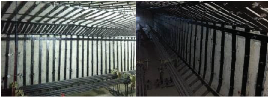
Figure 8: Steel plates on the interior of the girder web
