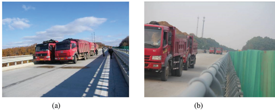
Figure 14: Eccentric loading of load test: (a) before strengthening; (b) after strengthening
