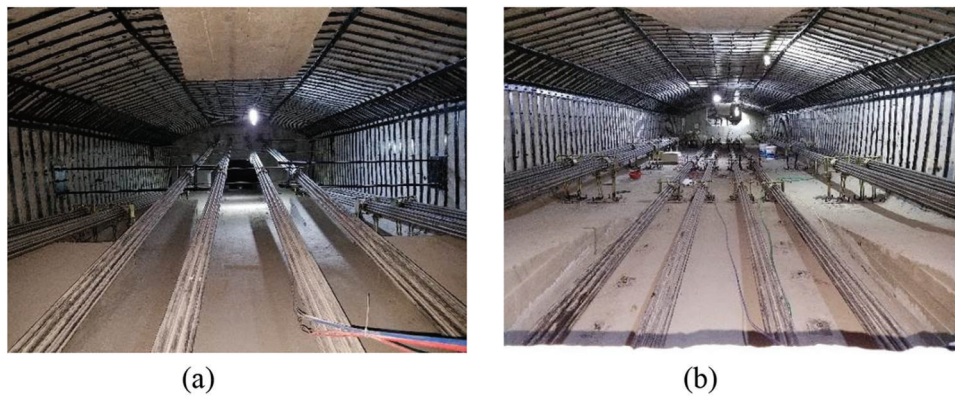
Figure 7: On-site installation of external prestressing tendon
