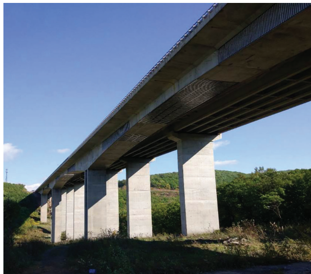
Figure 1: General view of the rehabilitated highway bridge
