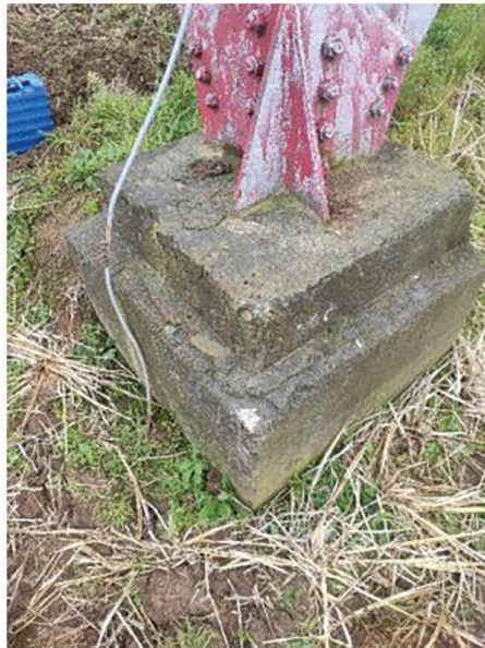
(a) Column A foundation
