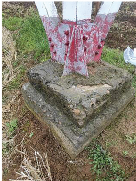
(c) Column C foundation
