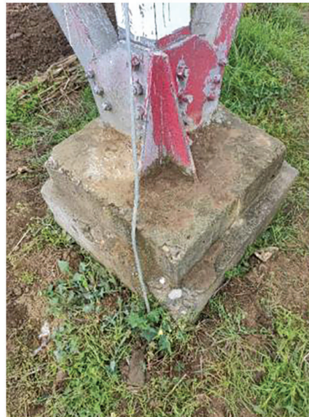
(b) Column B foundation
