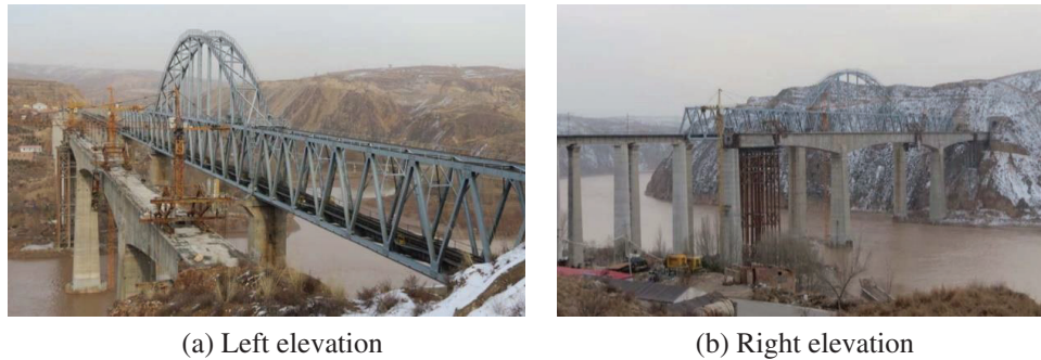
Figure 5: Overview of the main bridge of a super large bridge
