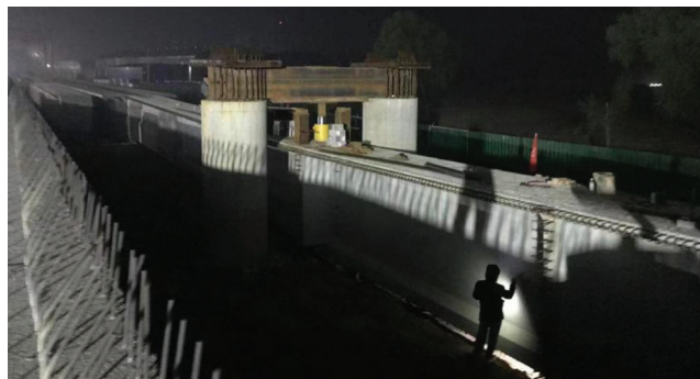
Figure 10: Field image of T-beam under load application
