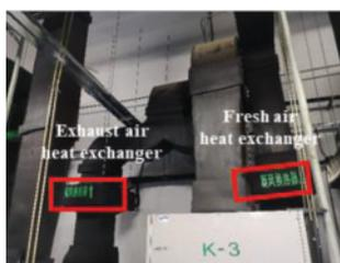
(a) MAHU-K3 and Fresh and Exhaust air heat exchangers of HRV
