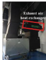
(b) Exhaust air heat exchanger of HRV-K1
