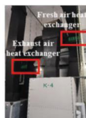
(b) MAHU-K4 and Fresh and Exhaust air heat exchangers of HRV
