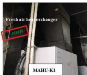
(a) MAHU-K1 and Fresh air heat exchanger of HRV-K1
