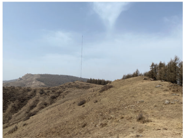
Figure 2: Anemometer tower on a complex topography
