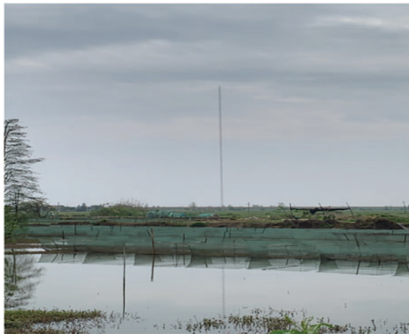
Figure 1: Anemometer tower on the plain topography
