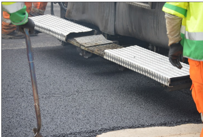
Figure 1: Laying the PASS at Alrewas Quarry.
