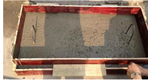
(a): Cast-in-situ concrete of the cement treated base
