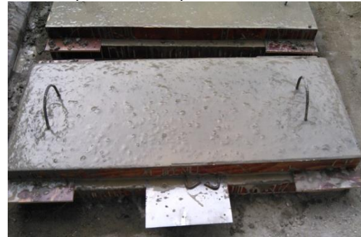
(c) Cast-in-situ concrete the track plate with precast crack
