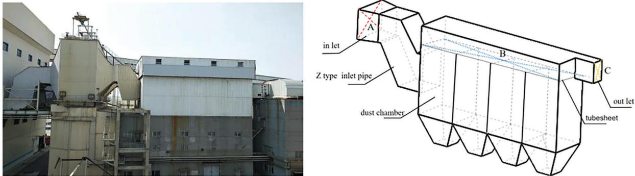
**Figure 1:** Appearance and model of the bag filter
