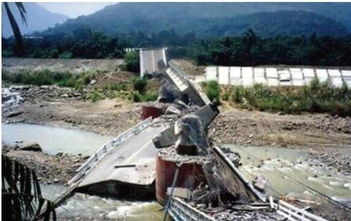
Figure 1: The Tong-Tou Bridge which collapsed in the Chi-Chi earthquake
