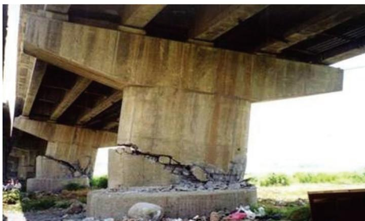
Figure 2: Shear failure of pier wall of the Wu-Shi Bridge in the Chi-Chi earthquake
