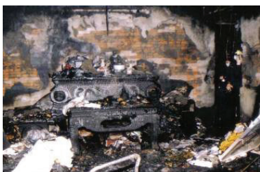
Figure 8: Interior furniture after accident
