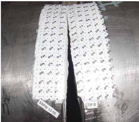
Figure 18: Pipe weld of 324 mm OD
