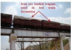
Figure 9: Formation of test train over the steel bridge considered in the present study
