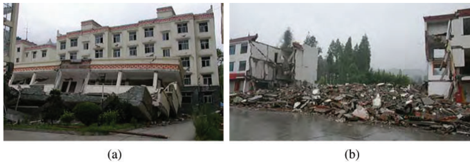
Figure 1: Structural damage and collapse during Wenchuan Earthquake, Sichuan Province, China, 2008 [6] (a) Collapsed four-story Xuankou Middle School in Yinxiu (b) The total collapse of buildings at Xiaoyudong due to Surface rupture
