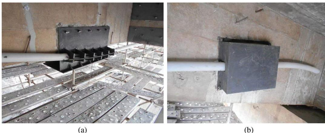
**Figure 10:** External prestressed reinforcement of main girder
