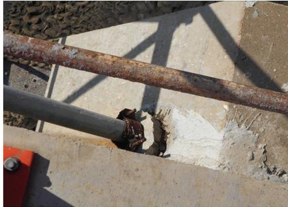
**Figure 6:** Cable anchor pulled out
