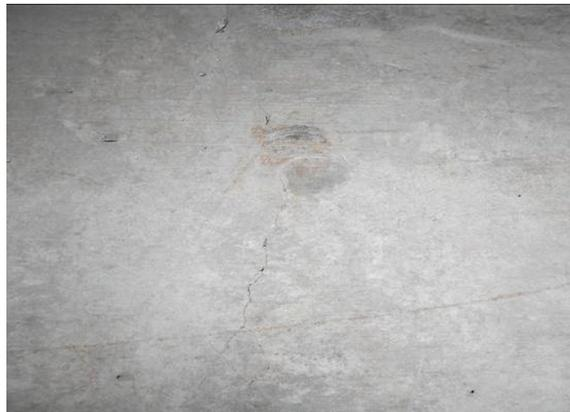
**Figure 4:** Oblique crack in main girder structure
