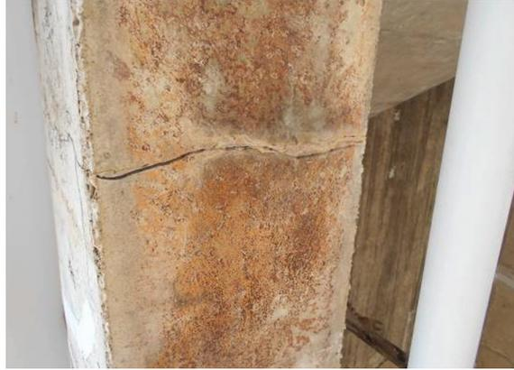
**Figure 3:** Vertical cracks in main girder structure
