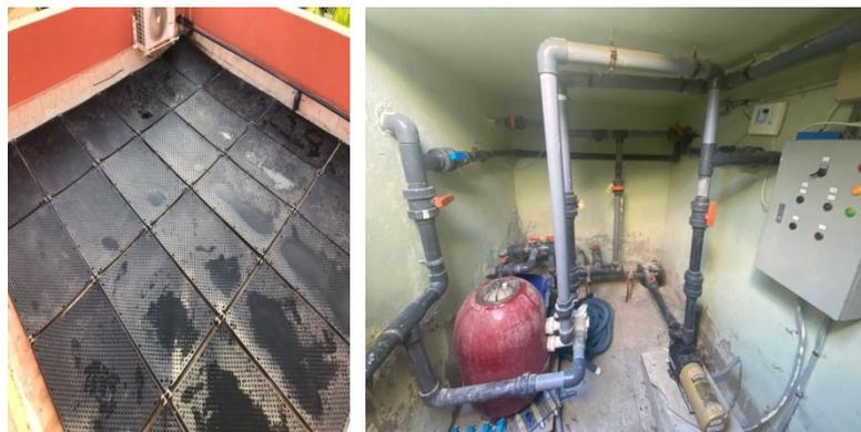
Fig. 14 SWHS proposed experimental scheme after components installed
