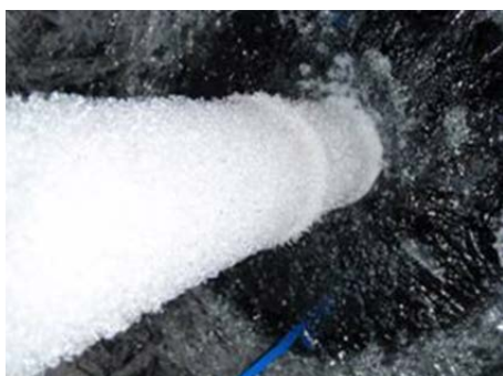
(b) Ice generation around the thermosyphon and inside ice storage tank
